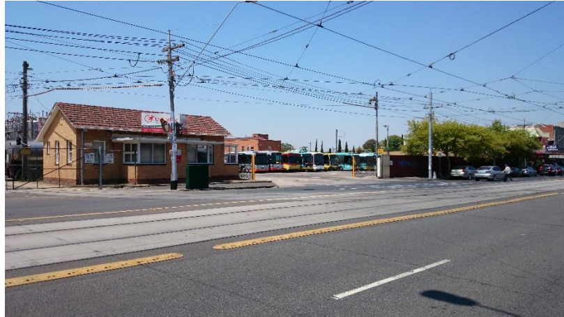
BUS DEPOTS FUEL & ELECTRICAL
