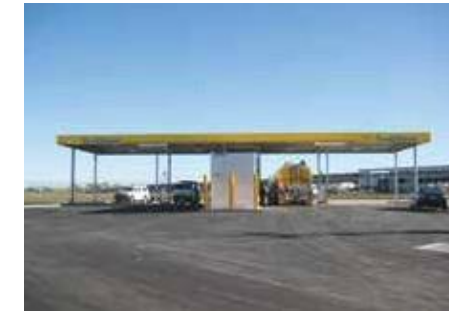
T80 & DGS : retail operation with bowsers positioned away from tank
