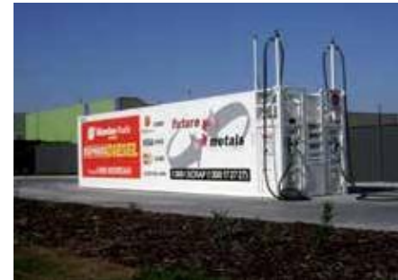
T68 : fitted with DCA and stand alone card acceptor
